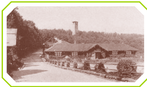
Electric Light Plant
